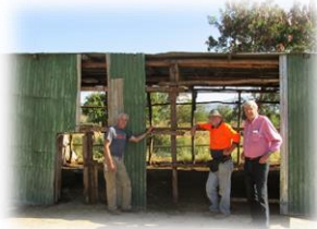
Goat shed under renovation.
